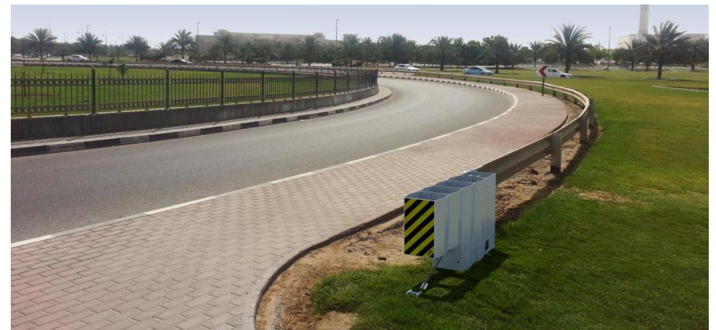
Simple and easy upgrade which provides robust anchoring for the guardrail and removes the potential for guardrail intrusion on impact.
