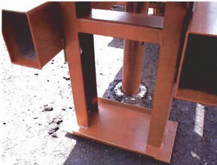
Figure 4 – Extractable tube inserted
