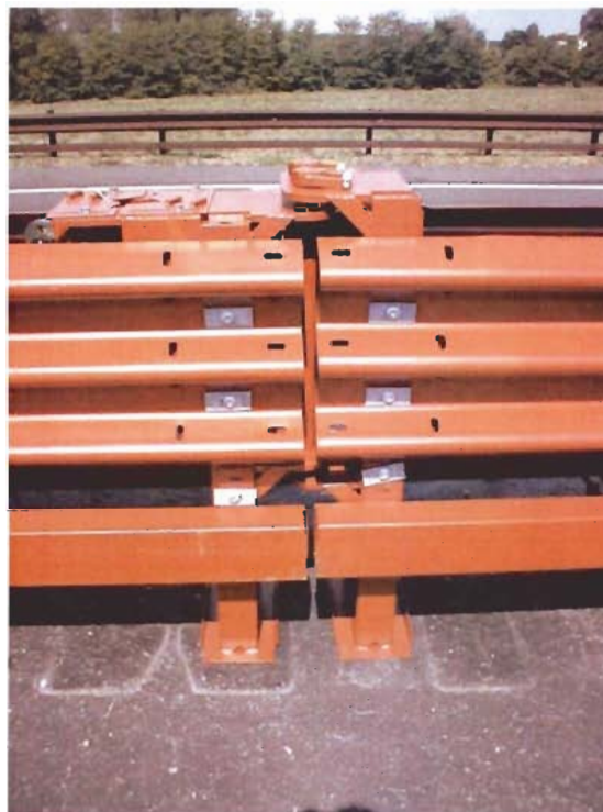
Figure 6 – SAB elements connected with pivots
