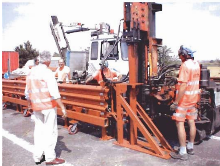
Figure 8 – Inserting of anchorage picket of backup support
