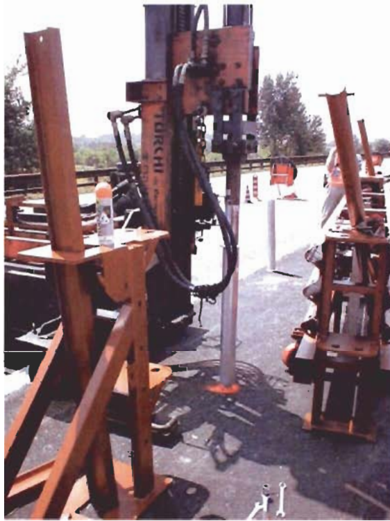
Figure 1 – Inserting of sleeve
